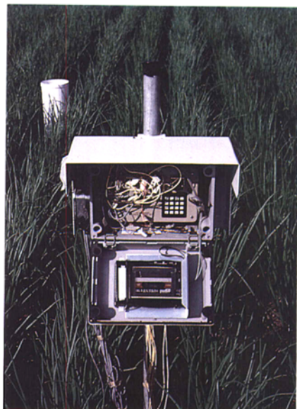
Fig. 13. Weather sensors and data-logging devices in an onion field. (Bottom) Data logger with nine input channels (Model CR-21, Campbell Scientific Inc.), positioned in a weather shelter.
