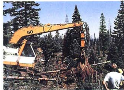
Fig. 6. Stump and root removal as part of site preparation before replanting in a forest affected by Armillaria root disease.
